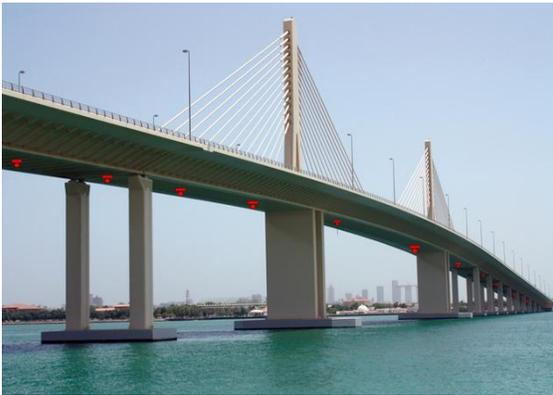
Fig. 8. Monitoring bridges using LWSN
