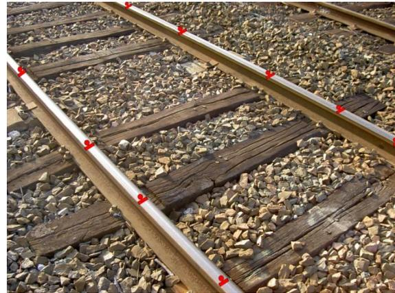
Fig. 5. Linear WSN on a railway
